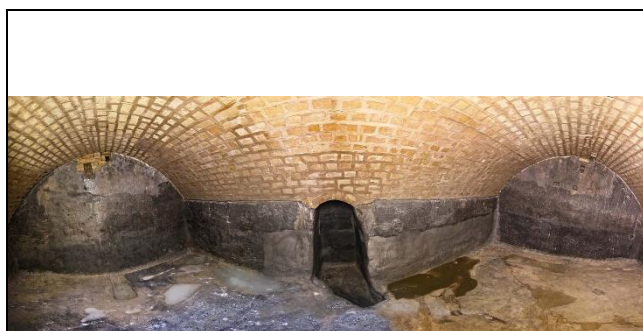
The Victory Square Reservoir following restoration
