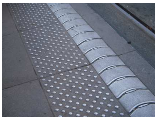
Detail of the tram stop.
