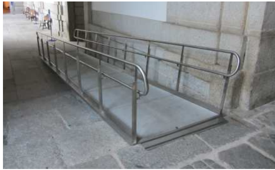
Ramp installed in Patio del Abrevadero.
