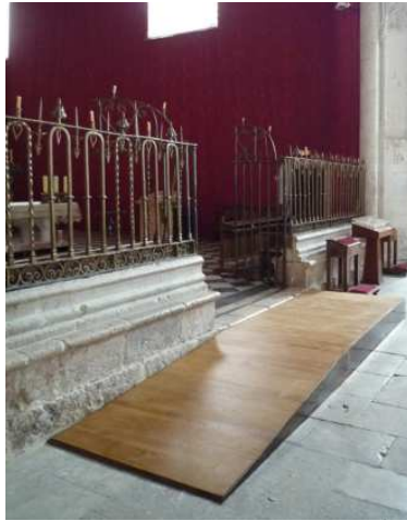
Ramp for access to the altar.
