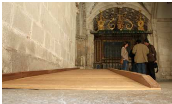
Non-slip ramp with lateral protection.
